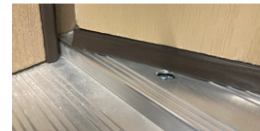
Inswing or outswing threshold mill finish
